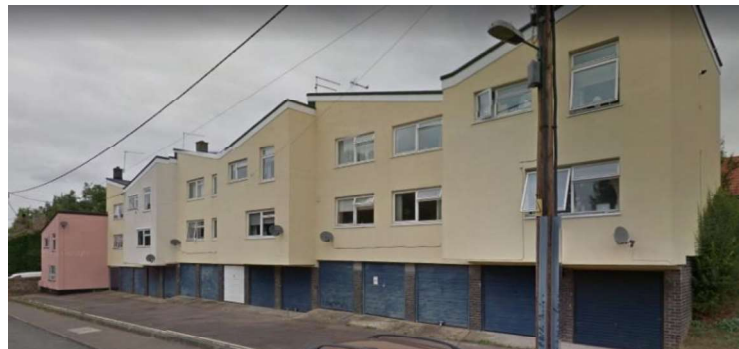
Thetford Road flats – lack of traditional materials used in design
