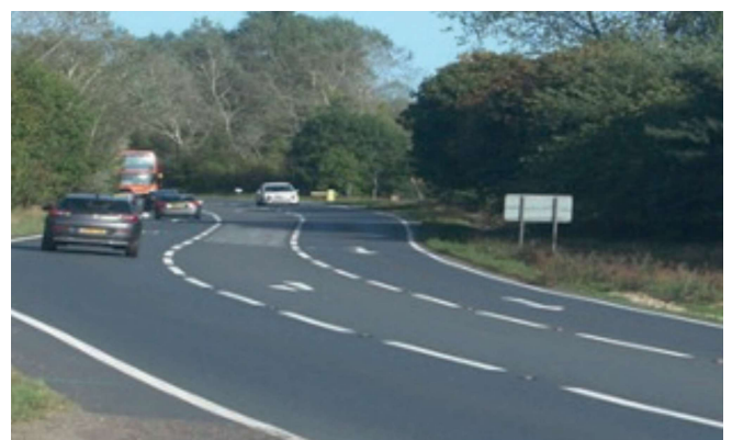
Ghost junction on Bypass
