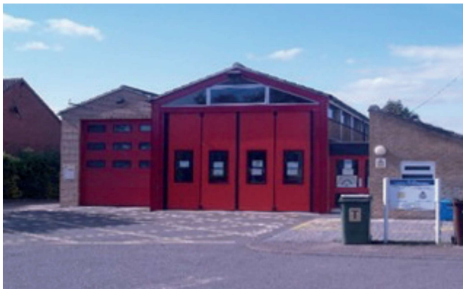
Ixworth Fire Station
