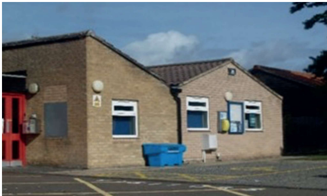
Ixworth Police Station
