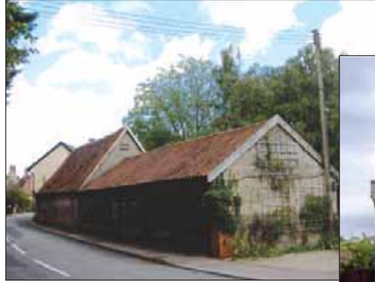
Photo 22: farm buildings in Bury Road
